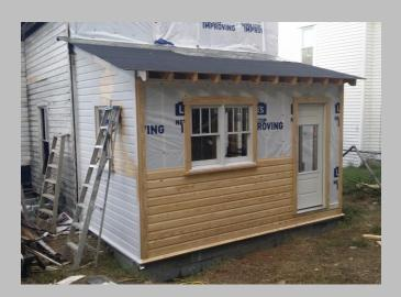
Due to a combination of poor framing and water damage, the rear porch that was enclosed in the 1930s needed to be razed and rebuilt from scratch, including pouring a new footing and foundation wall.
